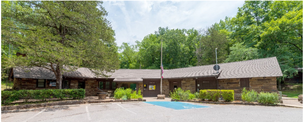
Figure 7: The current Visitor Center was built towards the end of the CCC period as part of a planned service group. The building now features asphalt shingles rather than its original oak shakes, as do most of the park's historic structures (Erdman, 2023).
