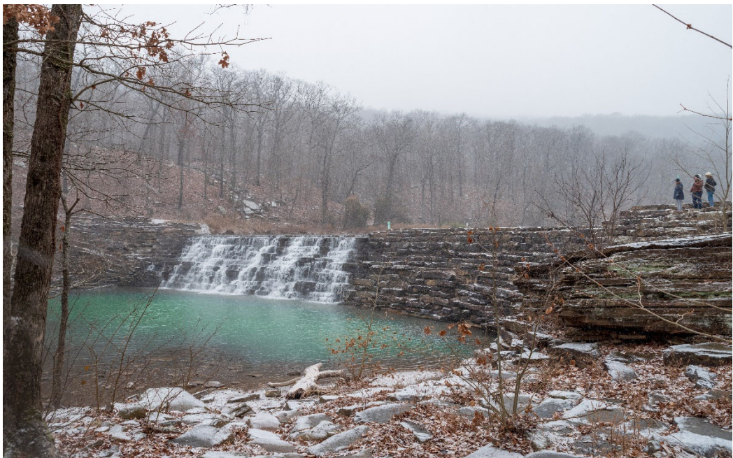
Figure 4: The CCC built a naturalistic stone dam on Lee Creek to create Lake Devil. The dam was raised two feet by Arkansas State Parks in 1972 (Erdman, 2022).
