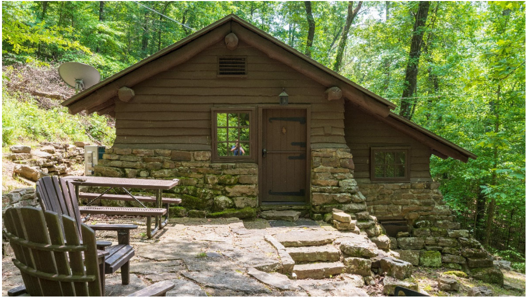
Figure 9: The park's CCC cabins employ a consistent design language but are highly varied in layout, size, and configuration. Cabin 16 is terraced into a steep slope (Erdman, 2023).
