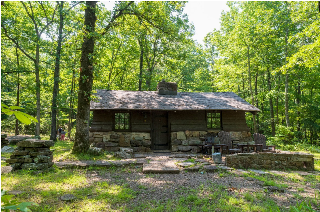
Figure 8: Cabin 6 sits in a forest clearing on a small knoll, largely secluded from its neighbors. Flagstone terraces and walks, stone walls, and stone lights that have been added to the park's original cabins since the CCC period are generally in keeping with the park's rustic style (Erdman, 2023).
