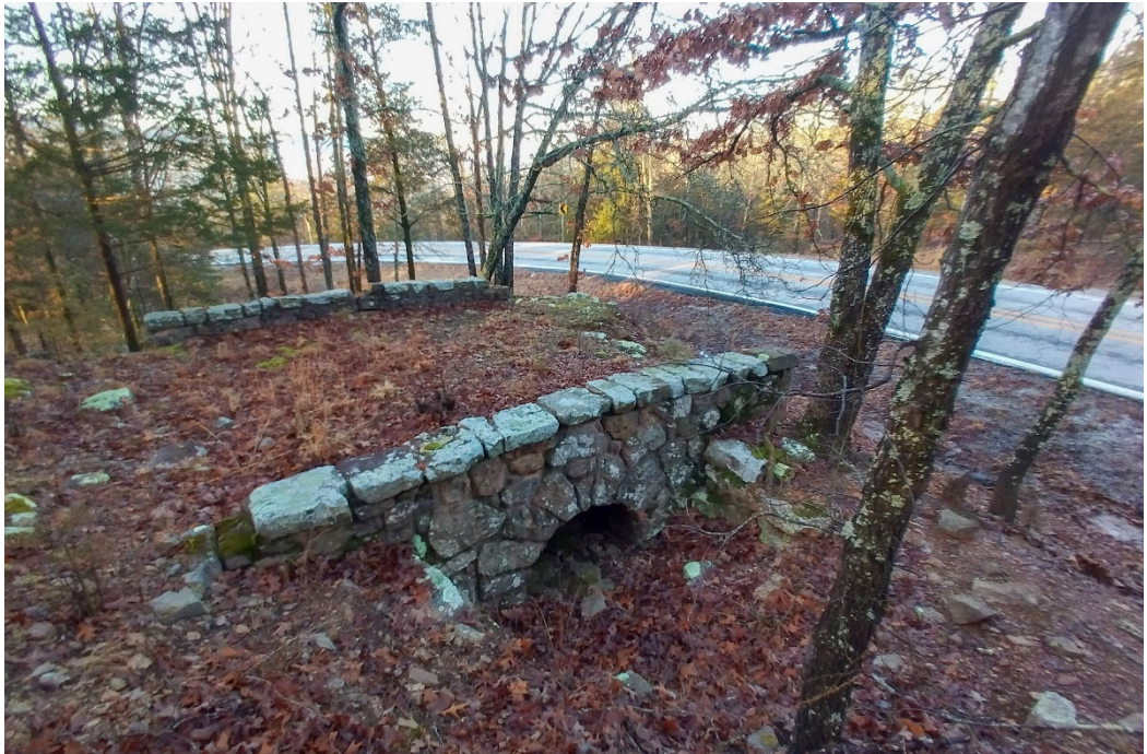
Figure 1: An abandoned CCC-built stone bridge on the former entrance road, portions of which were replaced by the new AR 170 (in background) in 1967 (Erdman, 2023).
