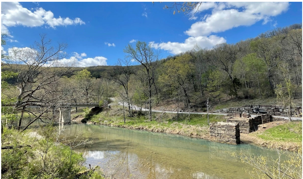
Figure 2: The original CCC bridge on AR 170 over Lee Creek was destroyed by a flood in 1959, leaving only remnants (right). The new bridge (left) built by ARDOT in 1960 did not follow the park's rustic design standards (Filbeck, 2023).
