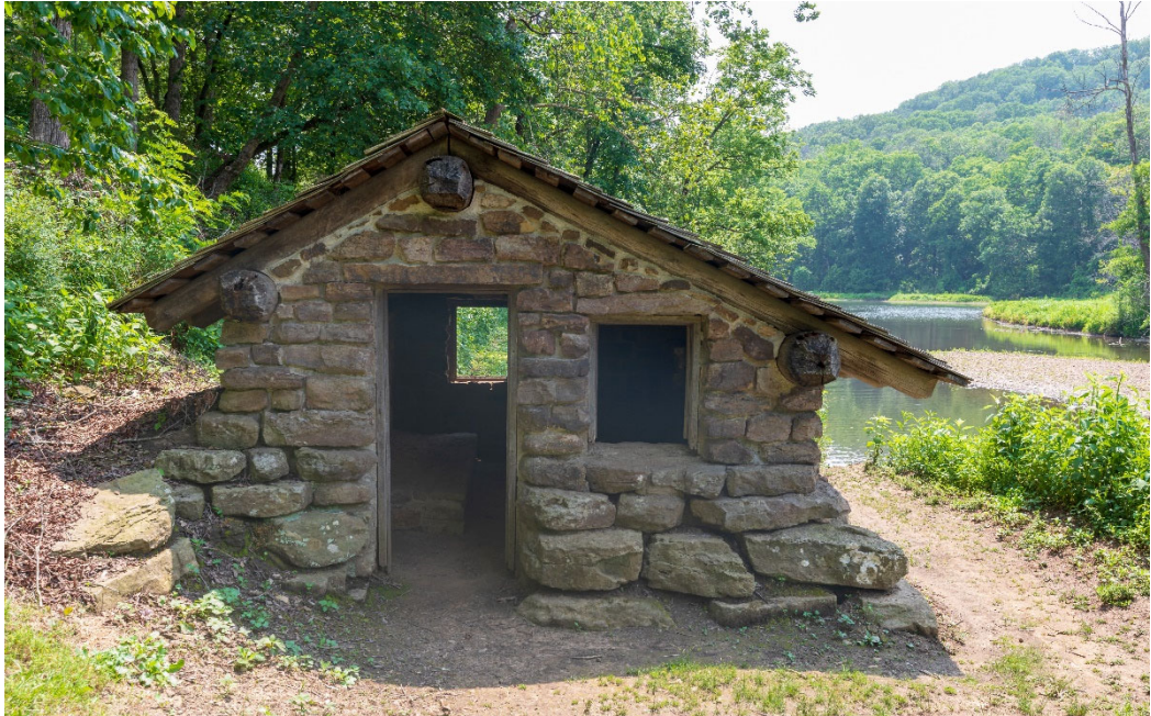
Figure 3: The CCC-built pump house on the shore of Lake Devil was restored by the Young Adult Conservation Corps in the early 1980s (Erdman, 2023).
